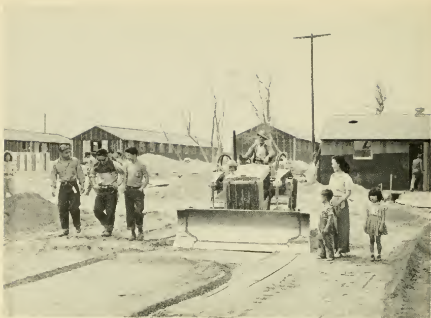
The contractor's equipment grades the streets at Manzanar while new arrivals watch.
