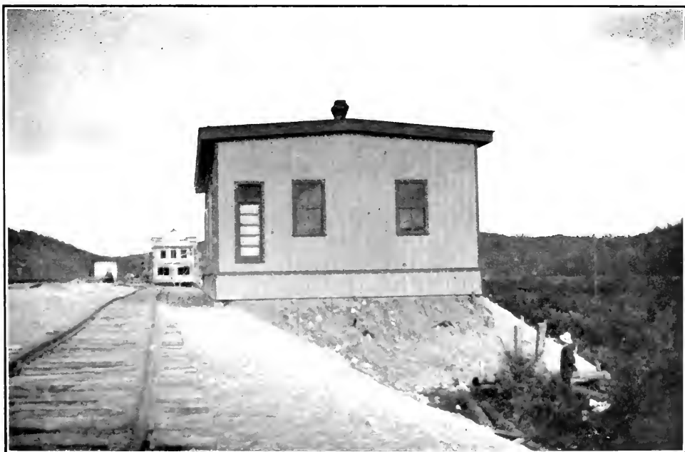
District F, Reddit. Freight Shed. Page 86
