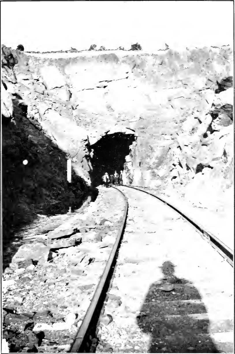
District A, Mileage 178.0. West Portal of Tunnel. Page 100.
