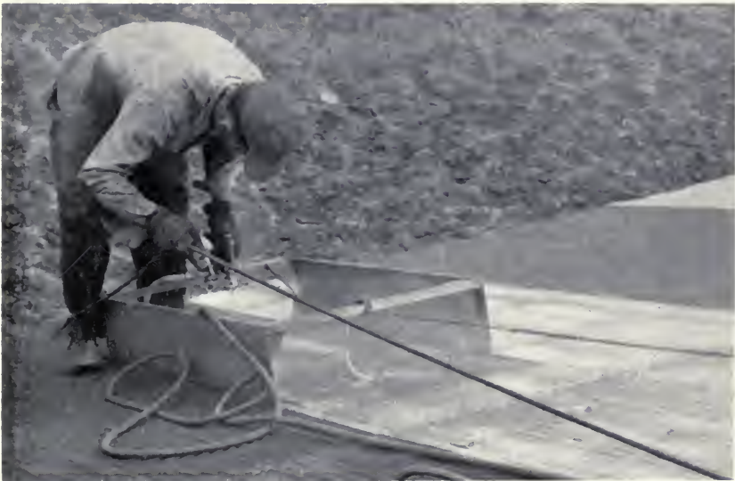
An aluminum shield was used to prevent spray from blowing to adjacent panels. (Fig. 3)
