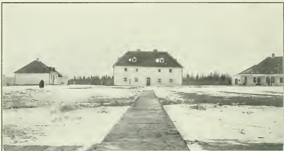
Norway House—From River Entrance.
